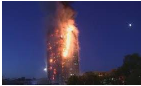
Grenfell Tower 14 July 2017, 80+ Dead or Missing
